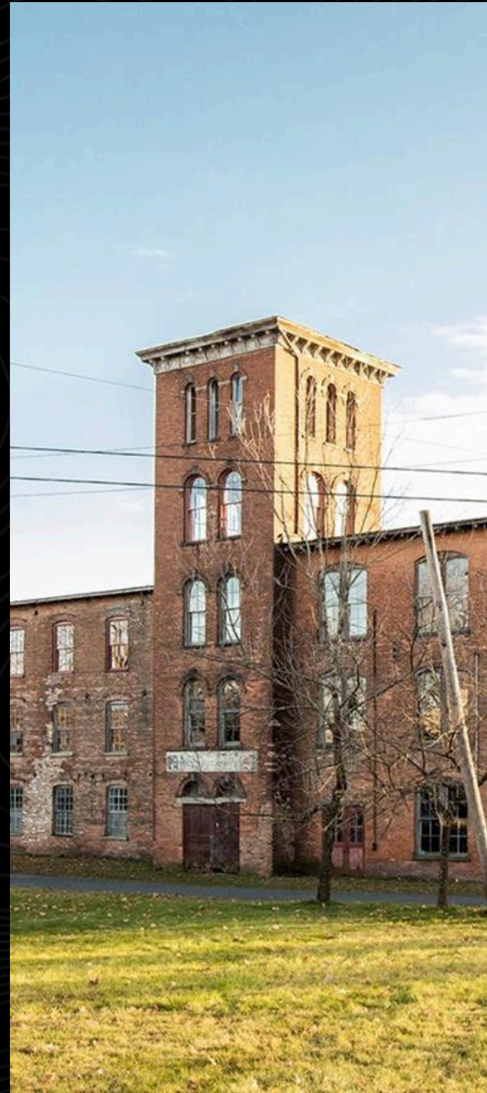
Summit Mill front entrance in its existing condition
